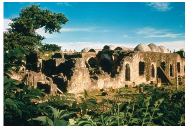
The Great Mosque at Kilwa , ca. 1100 C.E. The Swahili city of Kilwa, on the coast of present-day Tanzania, was likely founded by Muslim traders with strong links to the Indian Ocean world. The insides of its domes were lined with Chinese porcelain. Now in ruins, this large congregational mosque was probably in its day the largest fully enclosed structure in sub-Saharan Africa. How did trade across the Indian Ocean influence history in East Africa?
